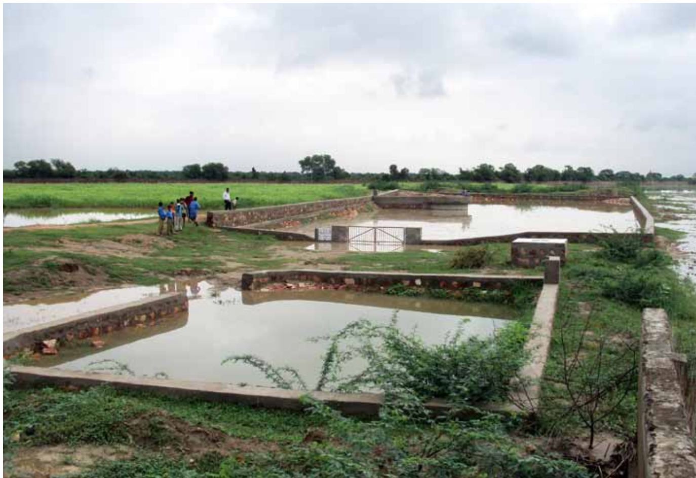
Collection of surface run-off water by the ponds made for groundwater recharging (Chak Ramnagar village, Bharatpur). RSNH Photo Library
