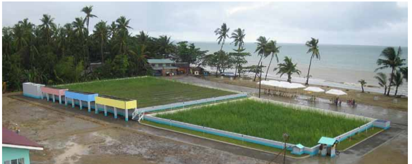
Constructed wetlands are a cost-effective wastewater treatment option, especially in per-urban and rural areas where land is available but capital may be a constraint. At Bayawan, a second-class component city, the local government raised funds to build and operate a reed-bed system in a coastal village. The treated wastewater is stored to supply water for gardens in the village and for fire-fighting. Steve Griffiths
