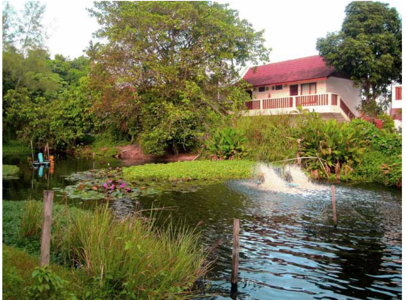
The wastewater treatment pond at the Frangipani Langkawi resort. Frangipani/Kuvinn Mallar Armugam
