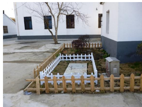
Figure 27. A PAWTP after installation
