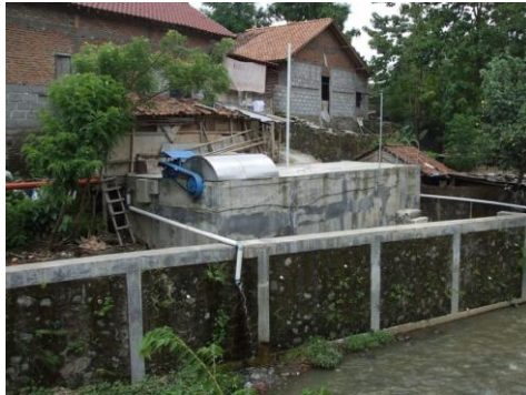
Figure 22. Model system in Karangwaru Dist., Yogyakarta City (Source: PUSTEKLIM)
