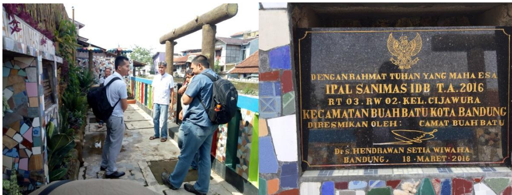
Figure 8. Example of anaerobic type DEWATS system (SANIMAS) installed and managed by a Community-Based Organization in Bandung, Indonesia (Source: Author)
