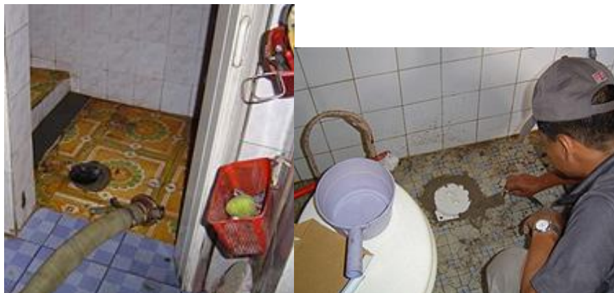
Figure 29. Worker installing a plastic cover to the access hole after septage emptying in Haiphong City (Source: 'URBAN DOMESTIC WASTEWATER MANAGEMENT IN VIETNAM', Water Environment Partnership in Asia)
