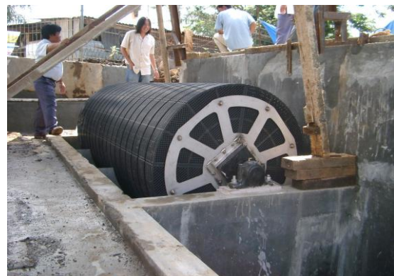
Figure 17. RBC with three-dimensional lattice contactors (Source: PUSTEKLIM)
