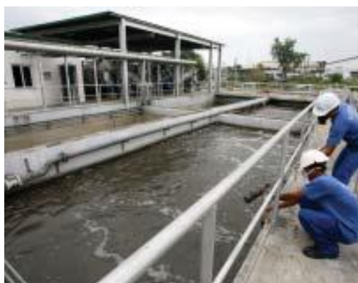
Figure 28. WWTP in Manila (Source: ADB CASE STUDY NOTES 'Septage Management')
