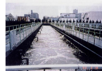
Activated Sludge Process
