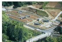
Oxidation Ditch
