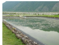
Wastewater Stabilization Pond (with Aerated Pond)
