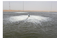
Wastewater Stabilization Pond (with Aerated Pond)
