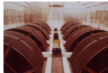
Rotating Biological Contactor
