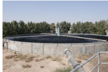
Trickling Filter
