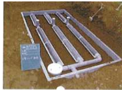
Figure T-13 Ground Treatment Tank
