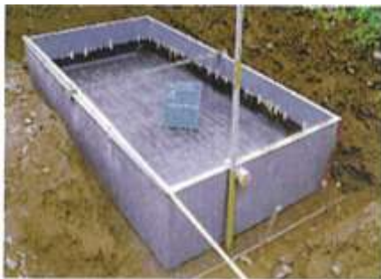
Figure T-12 Ground Treatment Tank
